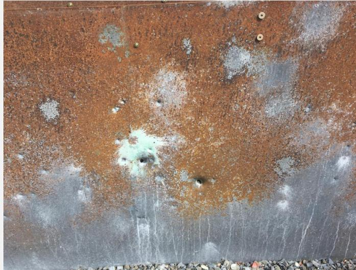
This is a picture of the plate designed to protect the trap house from being hit by incidental birdshot. This is not a target for testing slugs. This deliberate damage is uncalled for and causes range funds to be diverted to needless repairs instead of regular maintenance or expansion.
